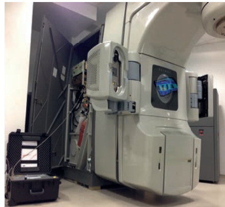
The B160R11 service unit is adapted to the requirements of small gas compartments. The photo shows the device during service works on an irradiation unit.
