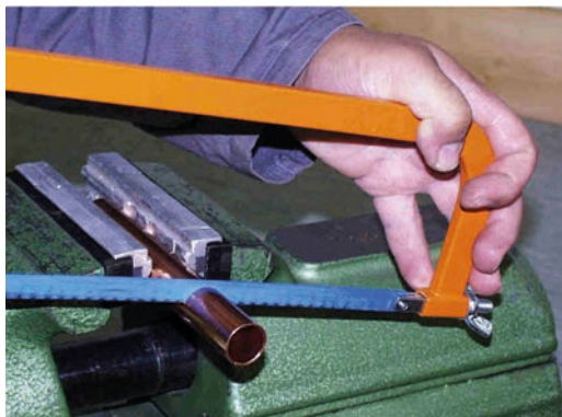
1. Rectangularly saw off the pipes
