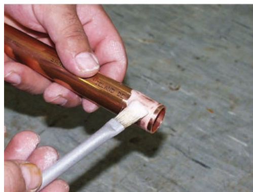
4. Apply the soldering flux on the pipe
