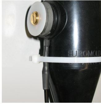
Fig. 4.3: Fixation with cable ties
